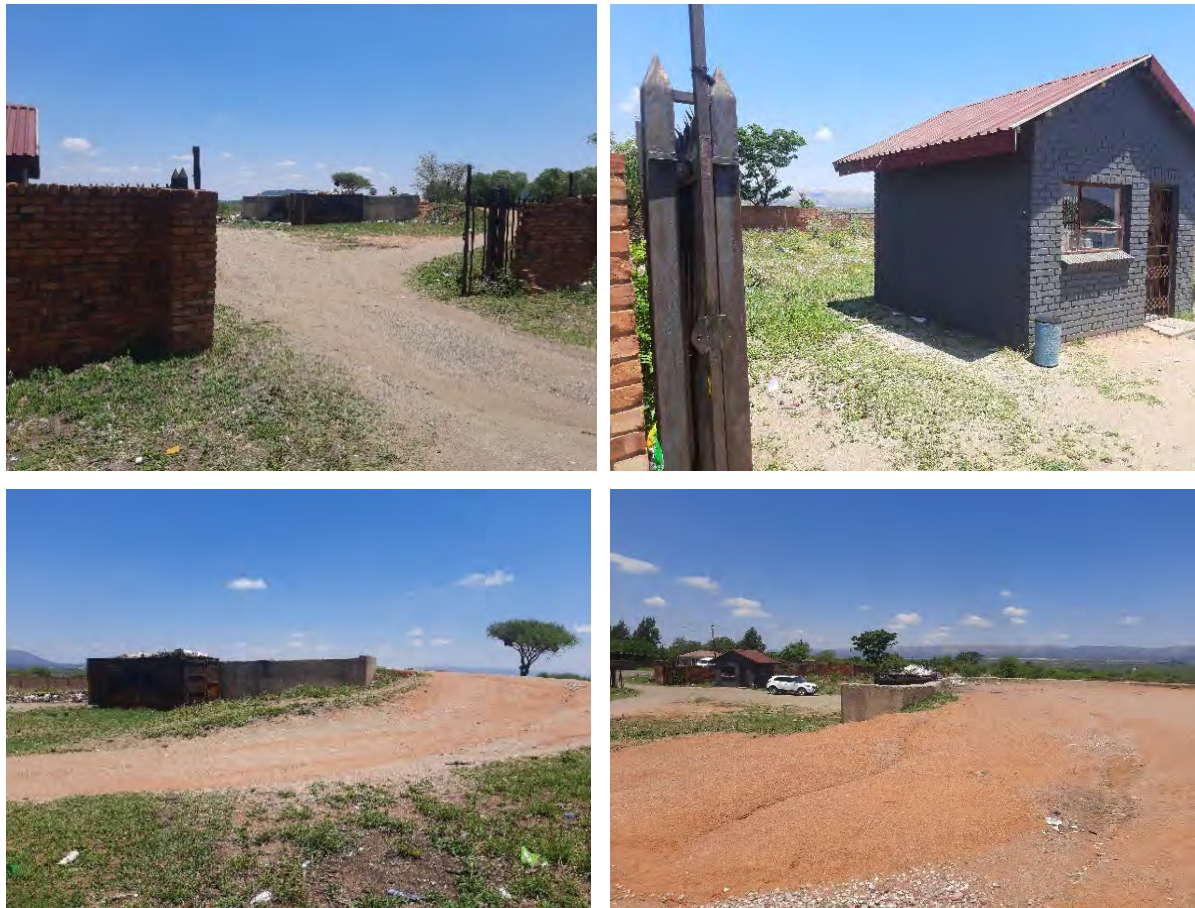
Figure 16: Mothotlung Transfer Station (09/11/2023)
