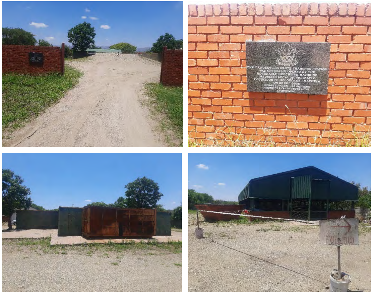
Figure 15: Damonsville Transfer Station (09/11/2023)
