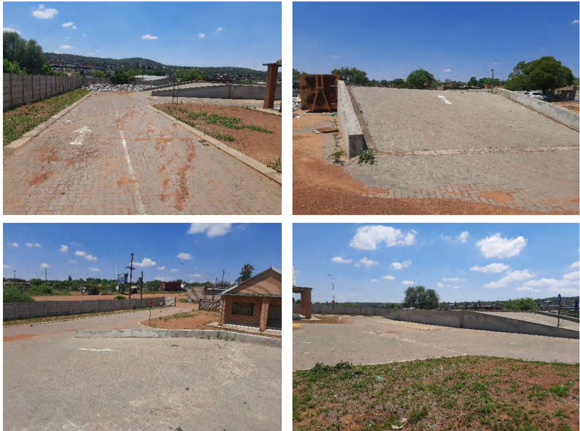
Figure 14: Hebron Transfer Station (09/11/2023)
